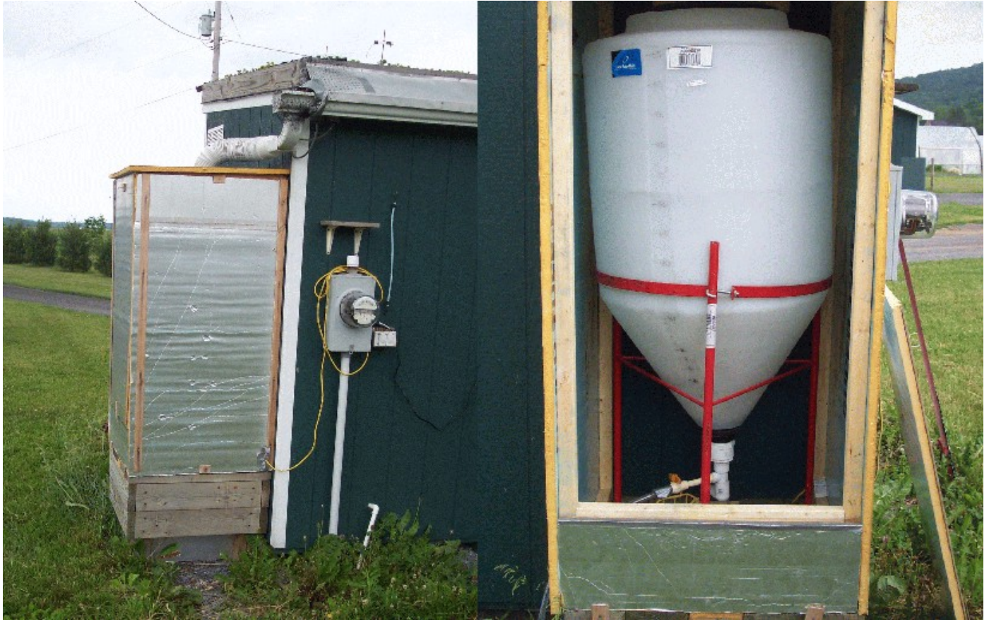
Figure A-6. Barrel enclosure with 1 in. (2.5 cm) insulation with a small heater inside to prevent the barrels from freezing (closed view on left and open view on right)
